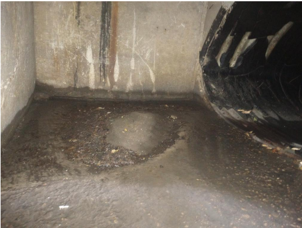
Photos of the transition from the box structure to twin CMPAs in structure AS4553-031.
