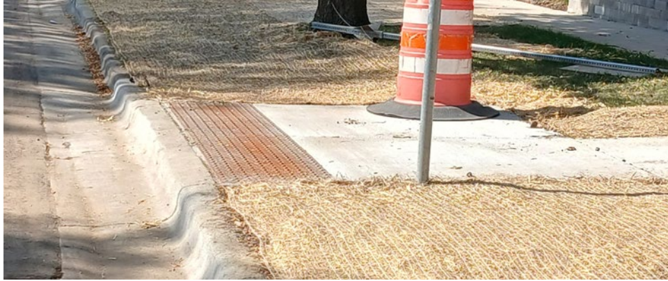
Raised curb head with detectable warning fields
