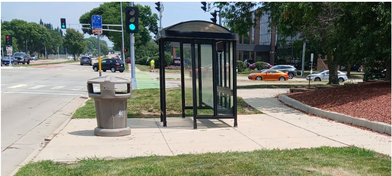
Sidewalk lowered with pedestrian curb
