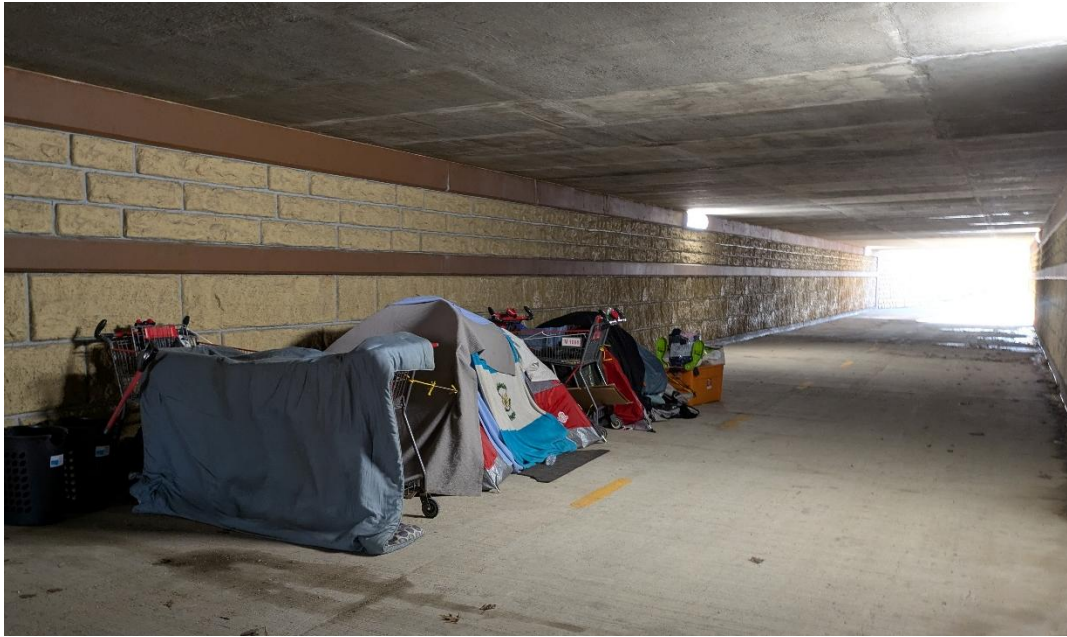
Figure 44 Encampment in the Gammon Road Underpass, April 9, 2026
