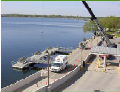
Law Park pier installation
