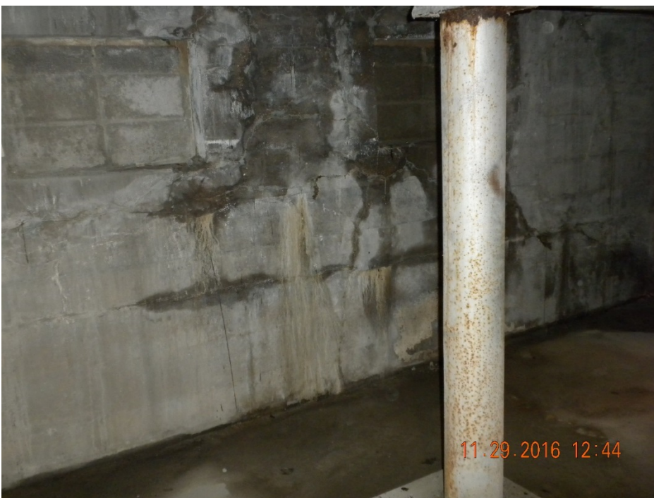
Moisture inside wall at North Dugout. Cracking in exterior wall membrane indicates this area is moving and is required to be stabilized once settlement cause is determined.
