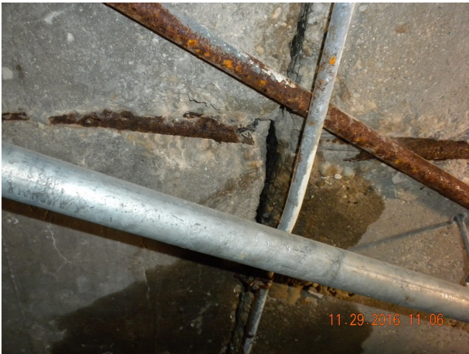
Water getting through the membrane at construction joint, causing damage to reinforcing steel and utility conduits.
