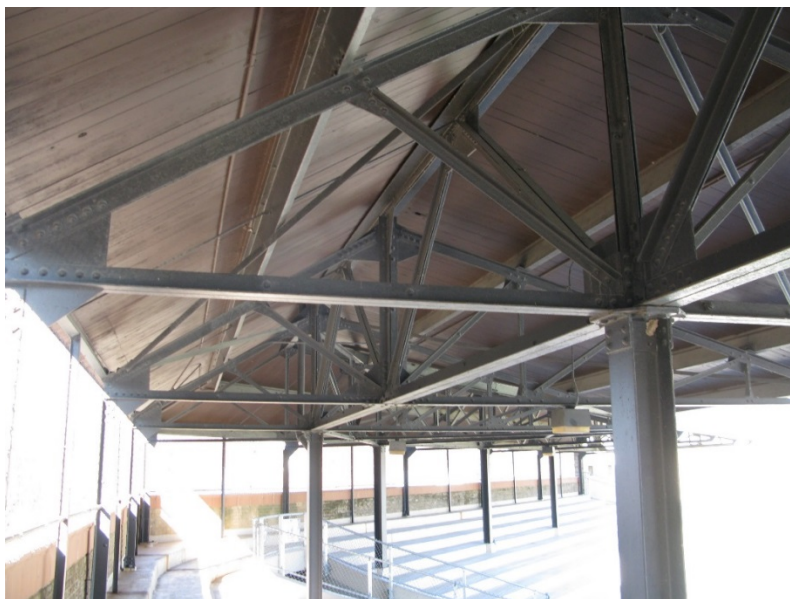
1925 Steel Truss Canopy
