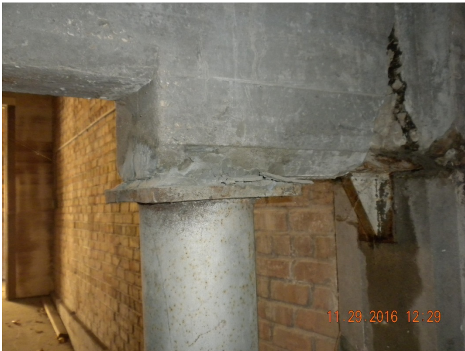
Previous damage to bearing end of concrete beam. Since supported. Support is adequate and in good condition.
