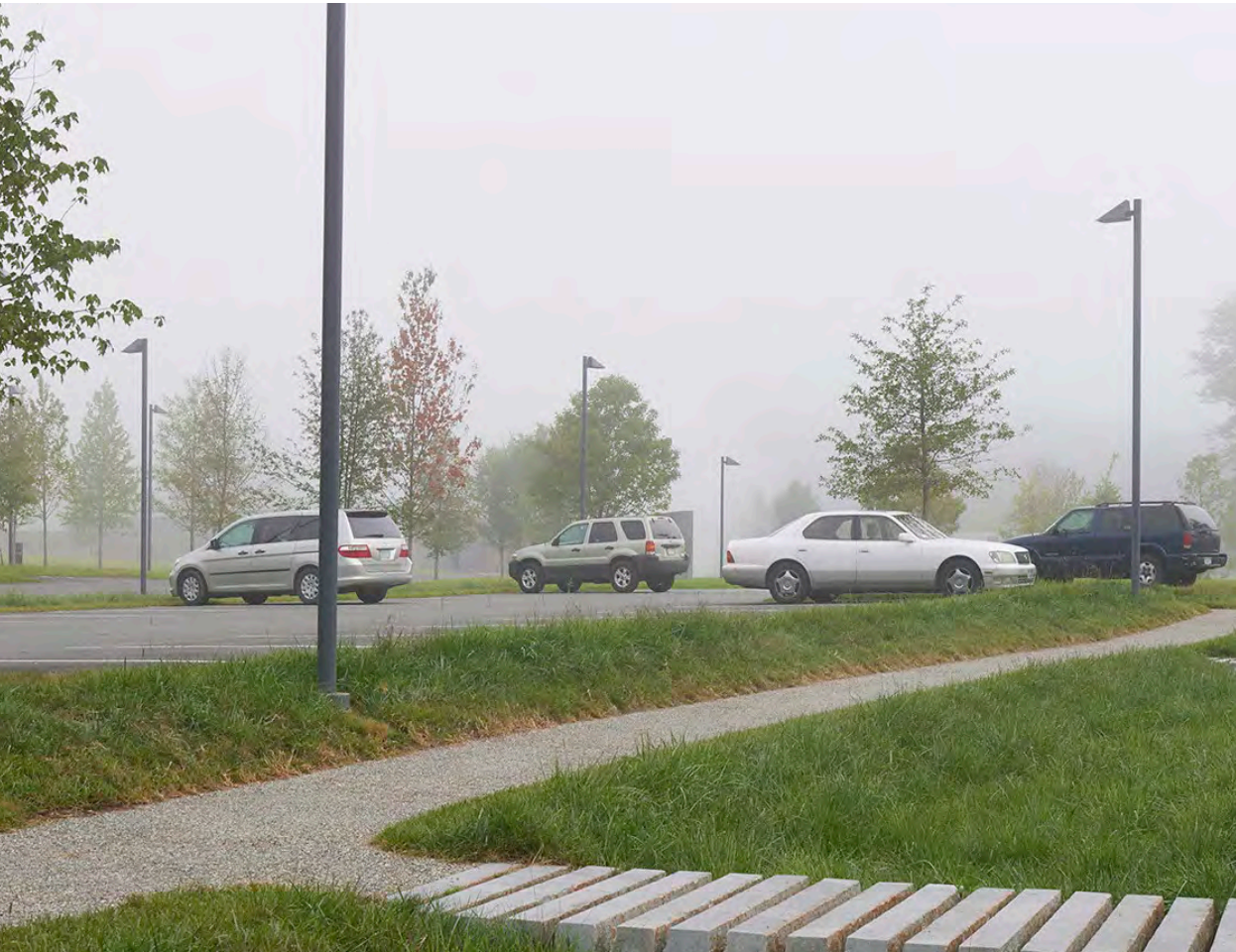
Stormwater treatment in the parking lot
