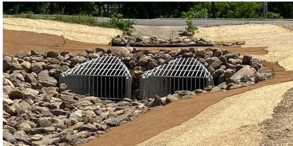
Example of dual pipe outlets
