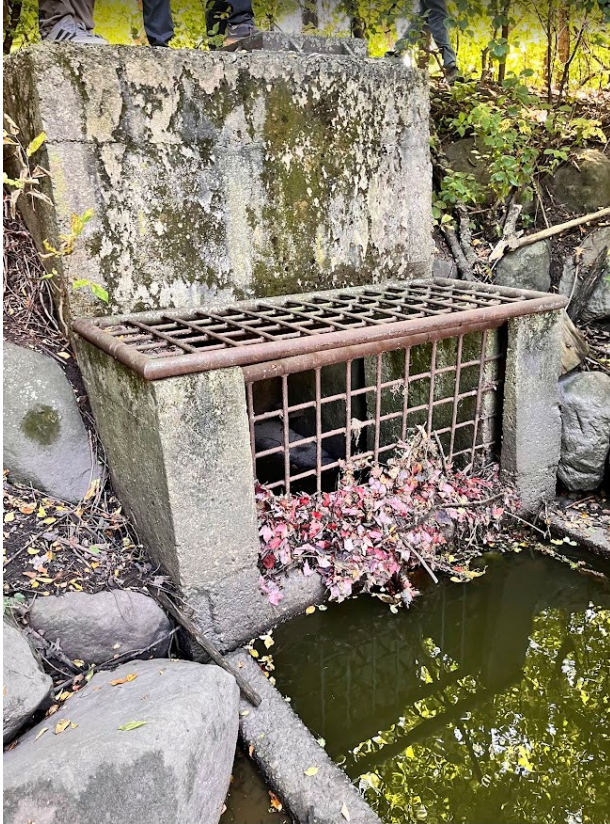
Existing control structure
