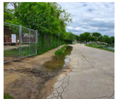
Figure 5.39. Slippage and Longitudinal
