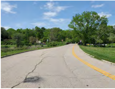
Figure 5.31. Longitudinal Cracks
