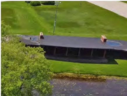
Figure 5.4. Water Ponding on Roof
