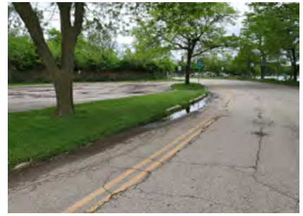
Figure 5.48. Drainage issues at South Lot
