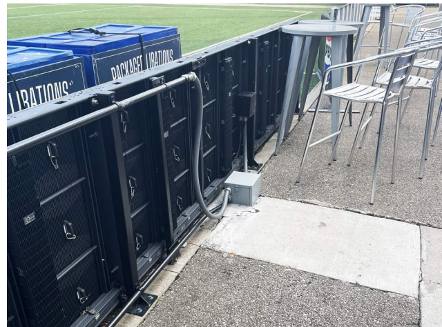
LED video boards line the eastern sideline. Mounted directly to a concrete curb; this creates a possible challenge during replacement.
