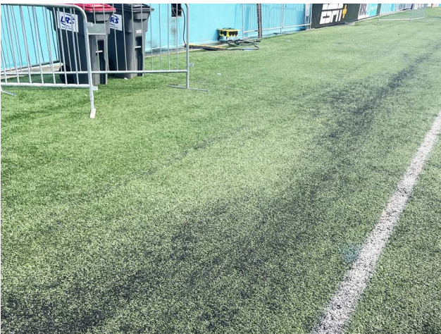
Excessive buildup of infill is evident along the boundary areas.
