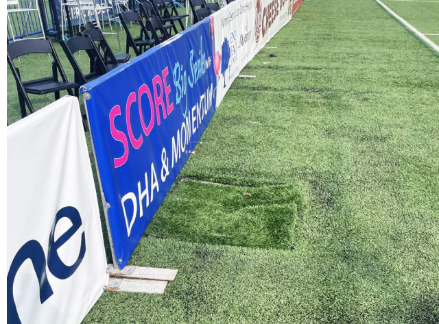
Removable patch of turf for goal post installation. The hatch cover is damaged and does not sit flush with the surface.
