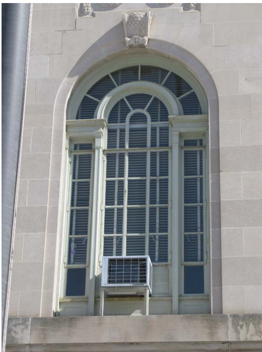
Figure 14 – Type W-2 Window with Four Operable Sashes
