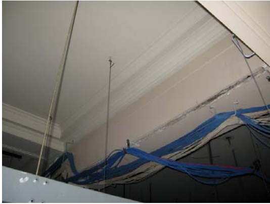
Figure 25 – Original Plaster Ceilings and Decorative Crown Moldings remain above the Suspended Ceilings on the First Floor
