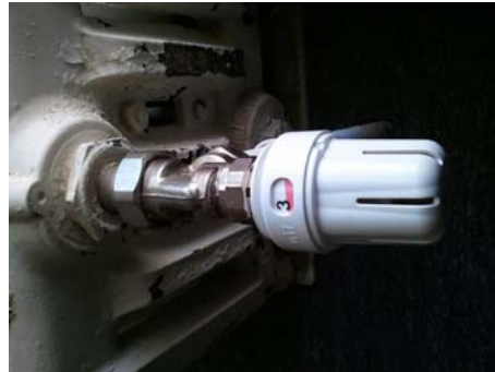
Figure 36 – Steam Radiator Control Valve
