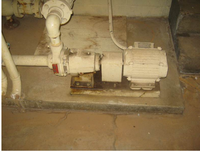
Figure 43 – Fire Pump
