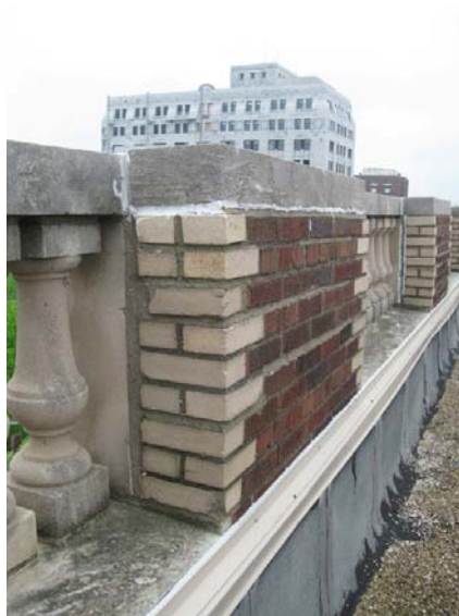
Figure 62 – Brick and Stone Parapet
