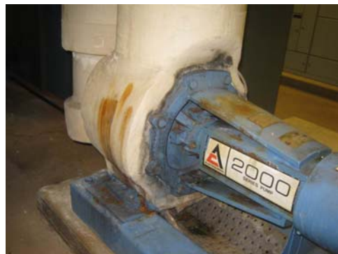
Figure 33 – Rust on Pump Header
