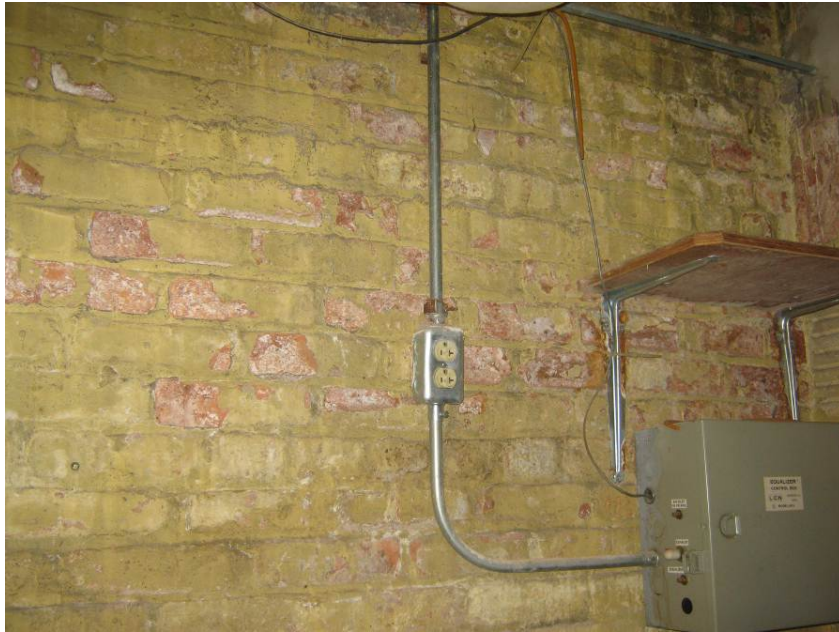
Figure 58 – Existing Brick Basement Wall Water Damage
