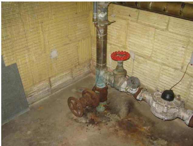
Figure 39 – Incoming Combined Plumbing and Fire Protection Service
