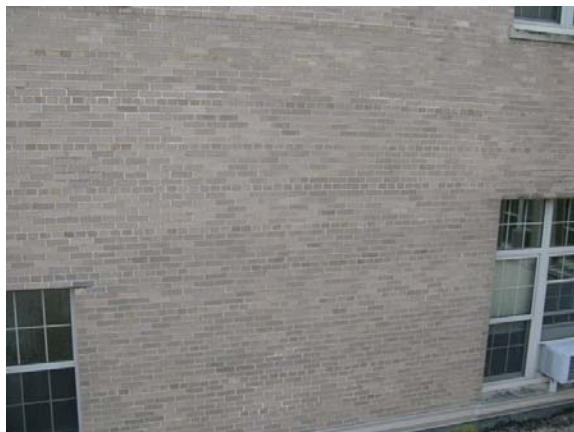
Figure 22 – Discoloration and Shifting of Brick indicates Rusting is occurring at the Hidden Relief Angles
