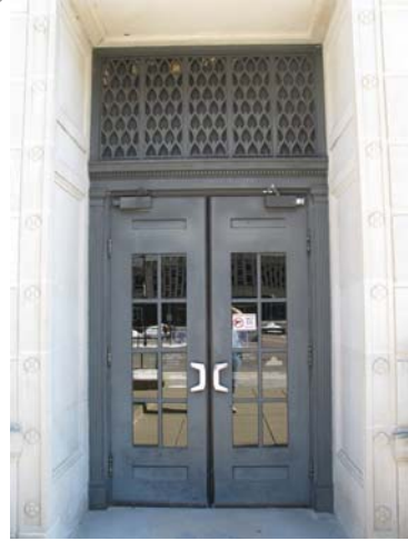
Figure 16 – Original Cast Iron and Steel Double Door and Transom Openings remain Intact
