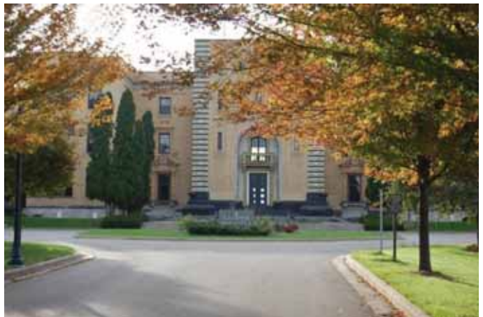
The High School Entrance
