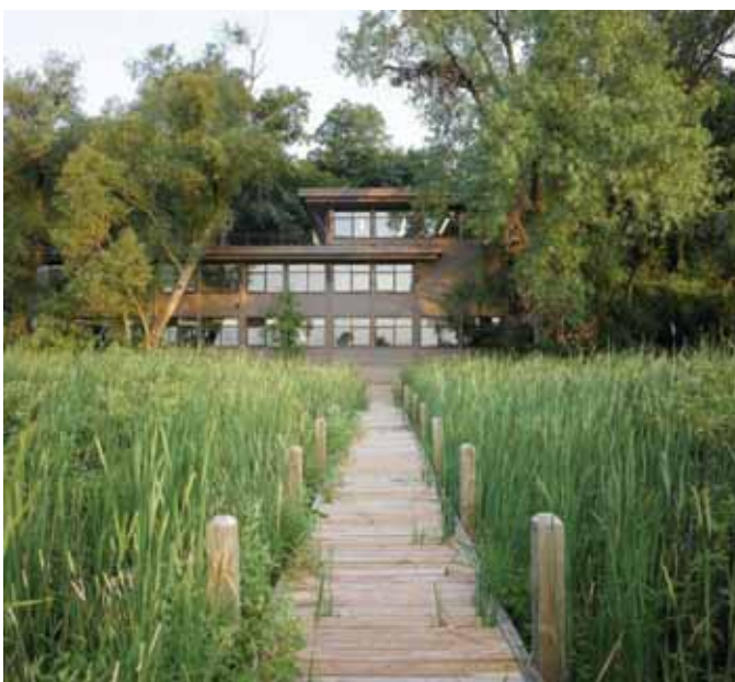
Wetland Boardwalk at Mazzuchelli Hall
