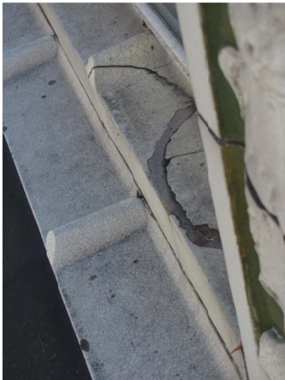
Figure 3. One cracked terra cotta window sill.
