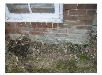
Patching the exterior foundation is an annual task as the winter ice/snow continues to deteriorate the foundation wall and undermine the brick above. Floor joists have settled with the house over years and interior floors are uneven making doors/windows difficult to close and maintain.
