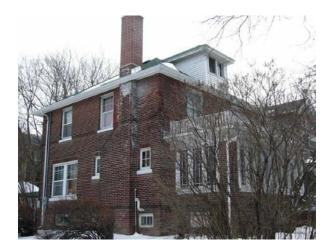
As you can see in this photo taken along Milton Street, the brick is heavily deteriorated and cracked from the chimney separating from the primary house structure.
