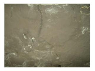
Close up of foundation cracking that is caulked annually due to increasing and additional deterioration.
