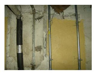
Photo is taken of basement foundation showing existing large cracks in limestone foundation wall that have been caulked. Existing piping has asbestos insulation covering original piping.
