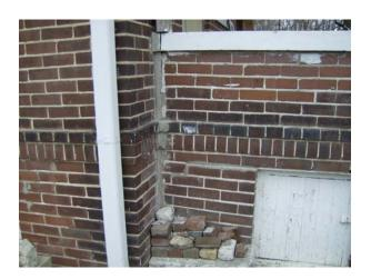
Shown in the photo is where the front porch connects to the main house. You can see that over the years, the porch has begun to separate structurally from the main house due to foundation settlement and cracking. The increasing gap has been filled with mortar, but continues to be a structural issue.
