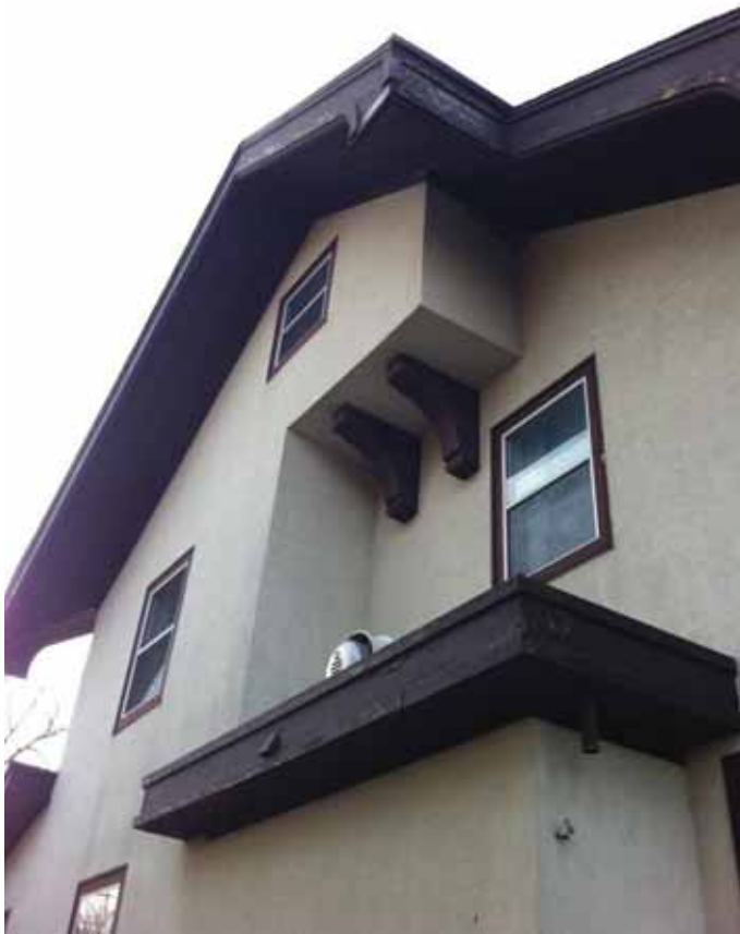
Figure 3 All exterior soffits are damaged beyond repair and the City of Madison correction order has not been acted upon. A dead squirrel fell out of the attic access hatch when we opened it because the damaged soffits act as squirrel entry points. It is difficult to see in photos, but the stucco is damaged here also.
