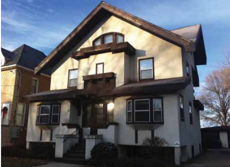
Figure 1 Primary view of house facing Sherman Ave. Significant degradation of soffits, gutters, stucco. The squirrels and raccoons enjoy the friendly confines of the roof thanks to all the holes. The stucco is not properly installed with rope and vee-groove. There is water damage behind the stucco as a result. The front bump-outs and rear additions were built without expansion joints and the stucco is cracking in these places also.
