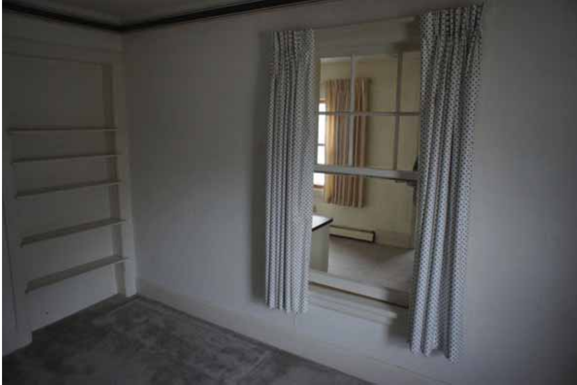
Figure 7 The three seasons porch was built in as an addition in the 1980's. Unfortunately, there are now disjoint spaces inside the house separated by formerly exterior walls and sliding windows. The entire second floor is also partially serviced by a live knob and tube circuit. The replacement electric panel is double tapped with loose connections throughout. This is a significant fire danger.
