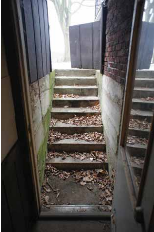
Figure 17 The 1980's remodel extended to the basement. While many thoughtful touches were added, they introduced new risks. For example, this sunk entry does not have any drainage (and has flooded into the basement repeatedly). Also, the foundation is cracked in this stairwell.
