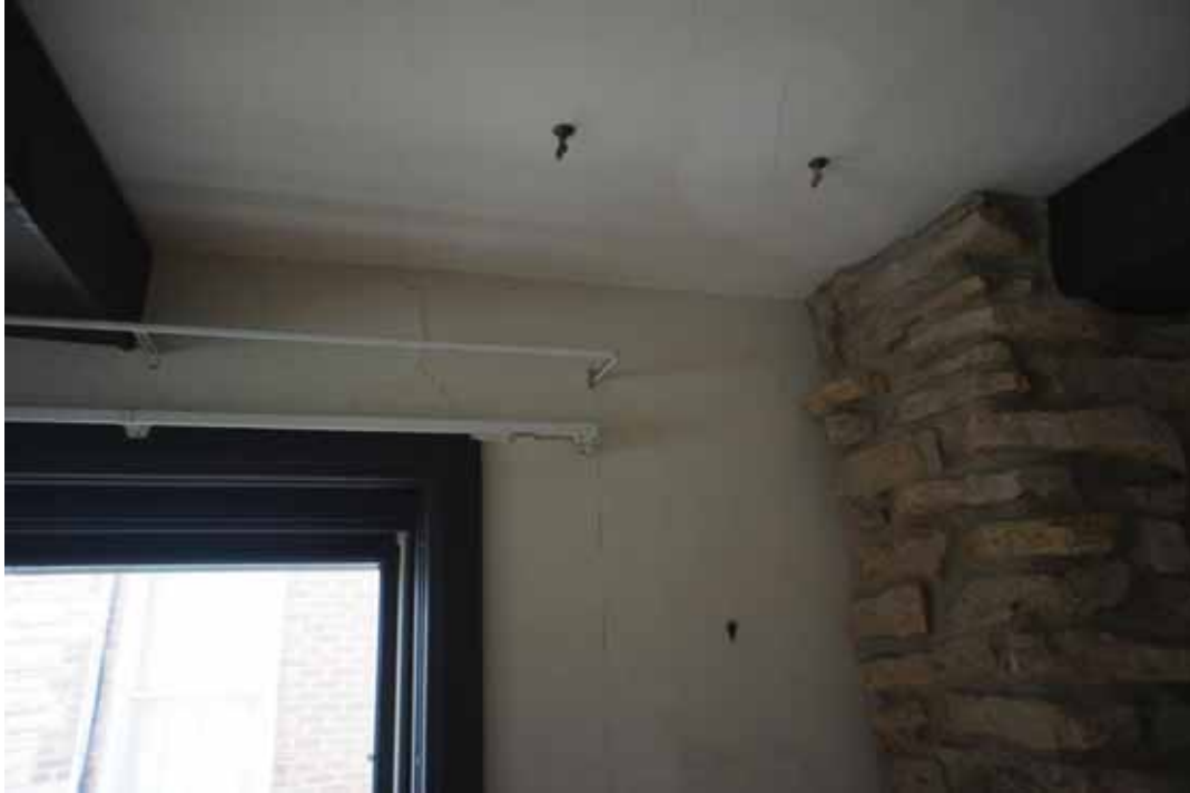
Figure 19 Water damage and plaster cracking around unoriginal ceiling beams and fireplace.
