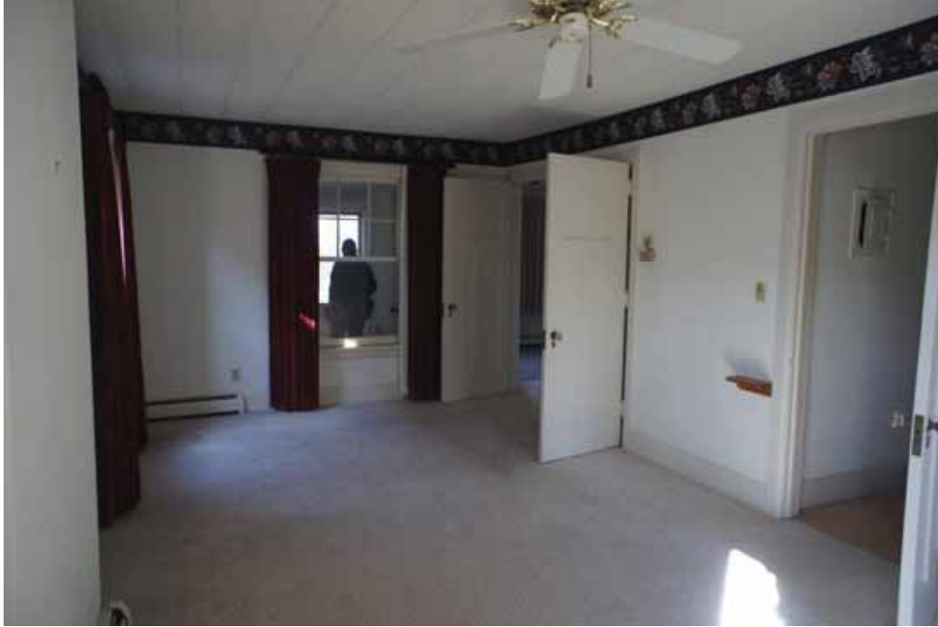
Figure 9 Dropped asbestos tile ceiling covering up original, water damaged, cracked plaster ceiling.
