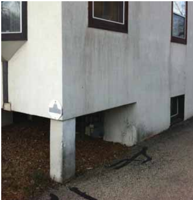
Figure 3 All exterior soffits are damaged beyond repair and the City of Madison correction order has not been acted upon. A dead squirrel fell out of the attic access hatch when we opened it because the damaged soffits act as squirrel entry points. It is difficult to see in photos, but the stucco is damaged here also.
