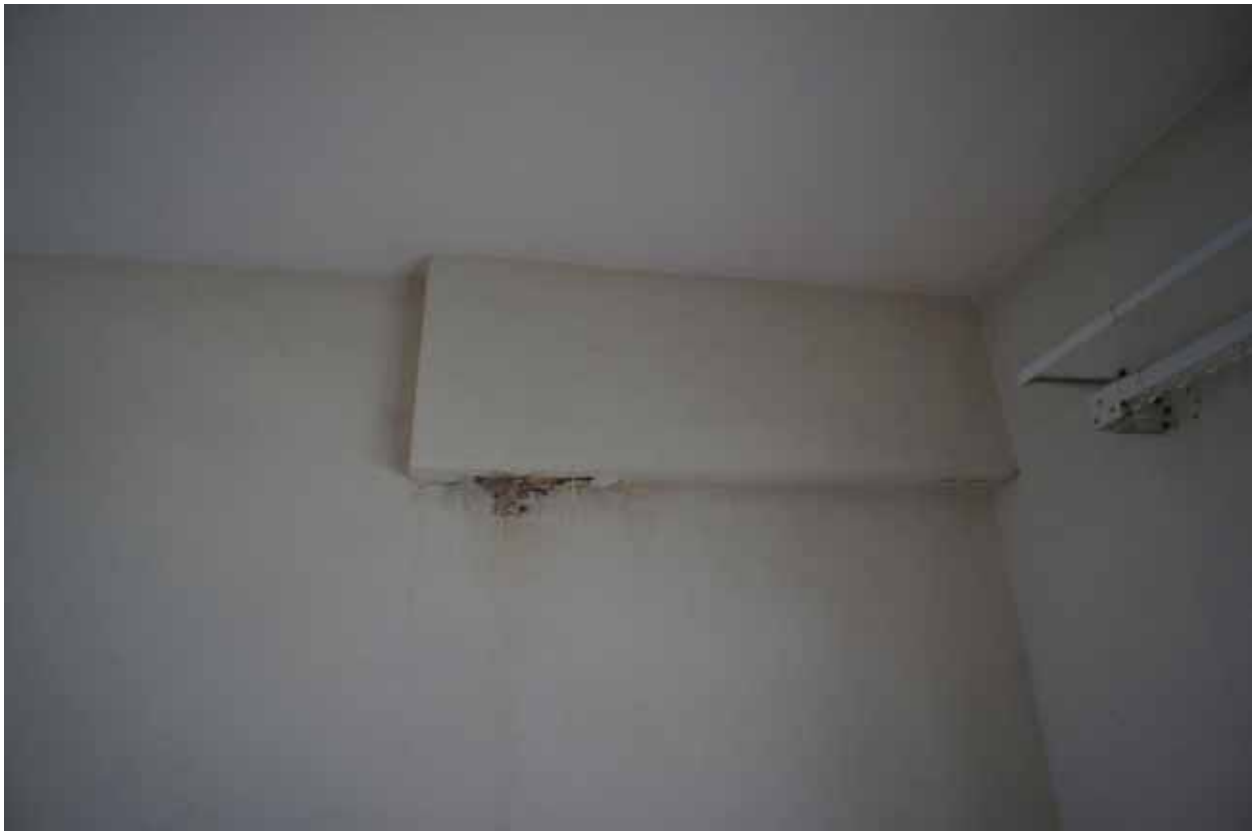
Figure 158 Water damage prevalent throughout (this is in the living room)
