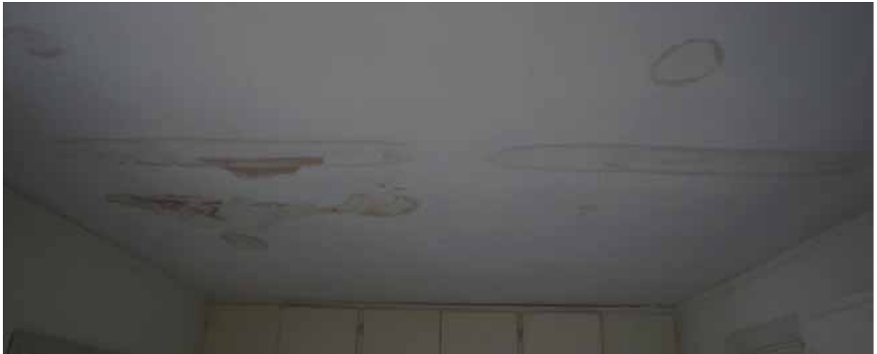
Figure 12 The roof over the addition is improperly drained and has been leaking through to the drywall below. Mold and water damage throughout.
