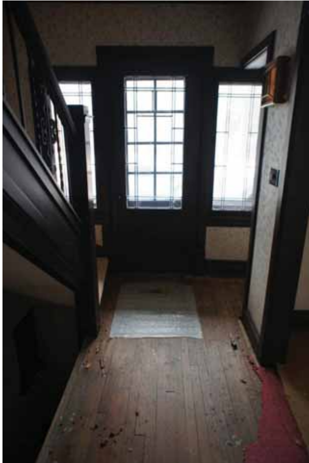
Figure 13 First Floor entry. Stairwell (and handrails) not as originally built. Existing wood floor was covered by carpet since last remodel, but is very damaged and has many missing pieces.
