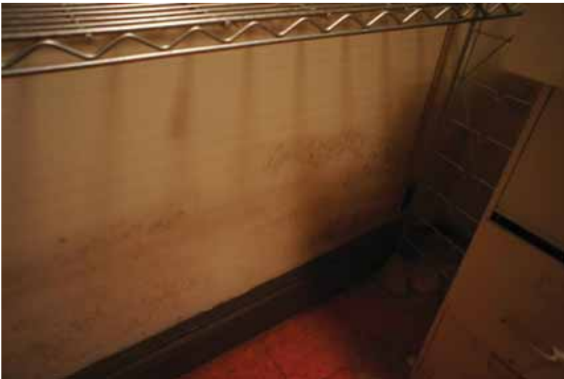
Figure 22 Mold has spread along the basement walls.
