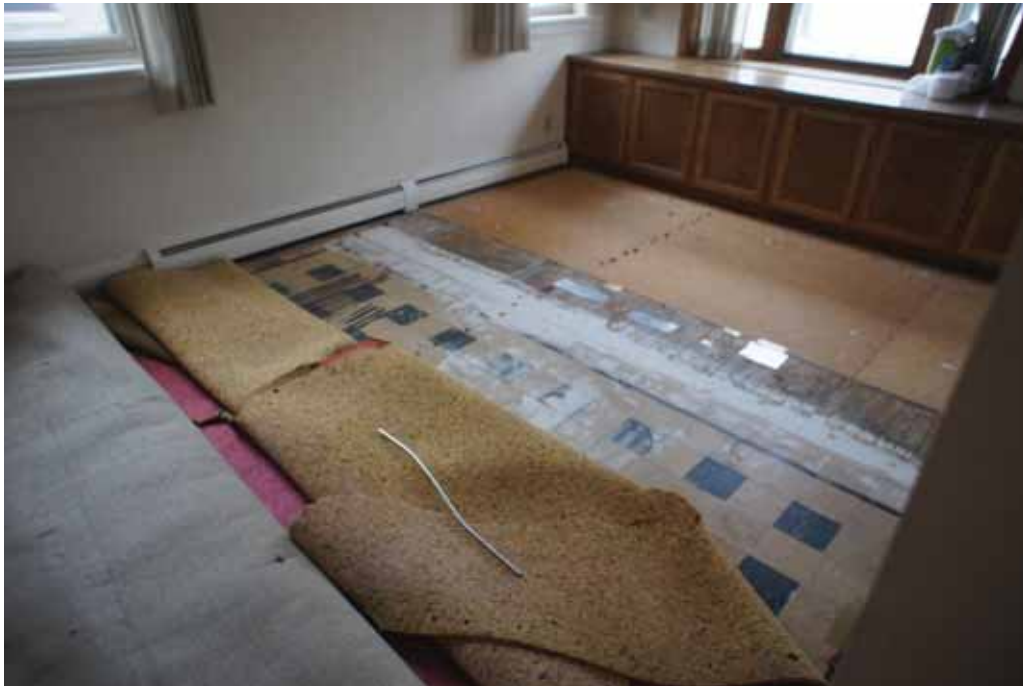
Figure 16 Dining room and living room extend into "bump outs" from 1980's remodeling. Walls are partially drywall and partially plaster. All trim and built in cabinets not original to house. Flooring is a mixture of asbestos containing tile, damaged wood and raw subfloor.
