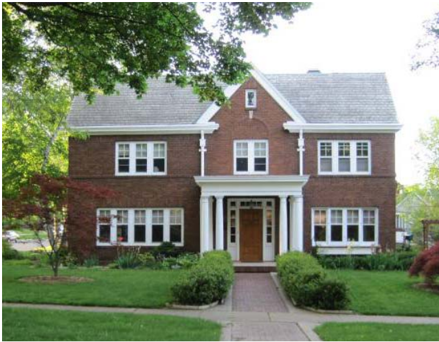
FIGURE 1. NORTH ELEVATION (FROM VILAS AVE)
