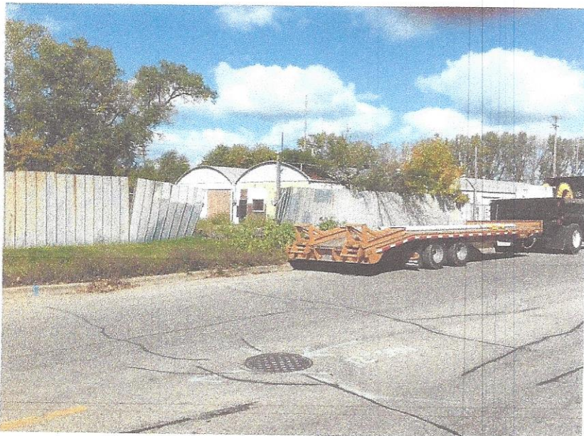
Street view through storm damaged, graffiti target metal fence, to be removed
