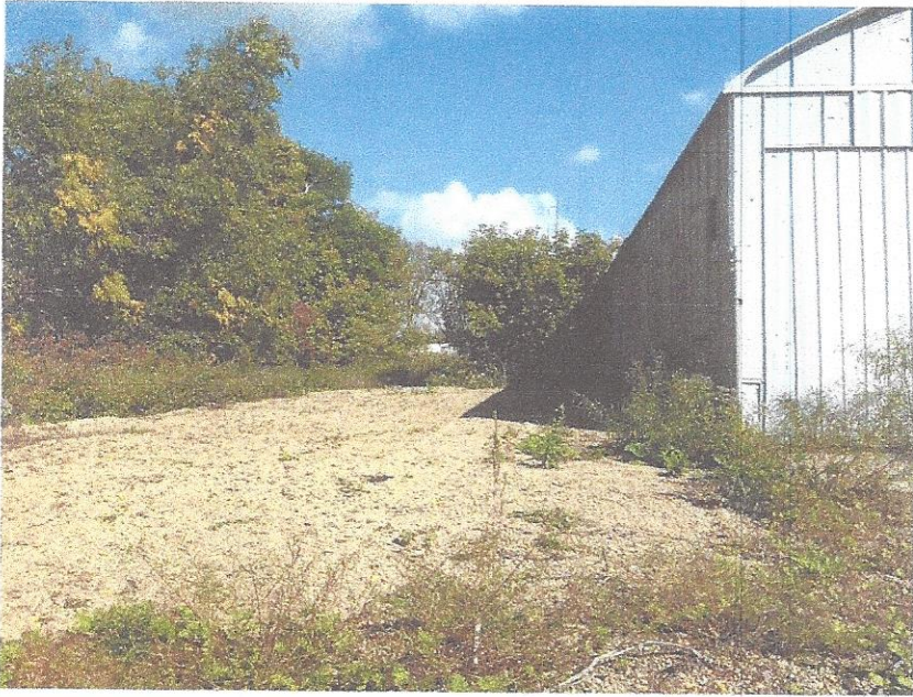
Gravel cap to remain on west side of building, view from south, facing north towards Sycamore Road
