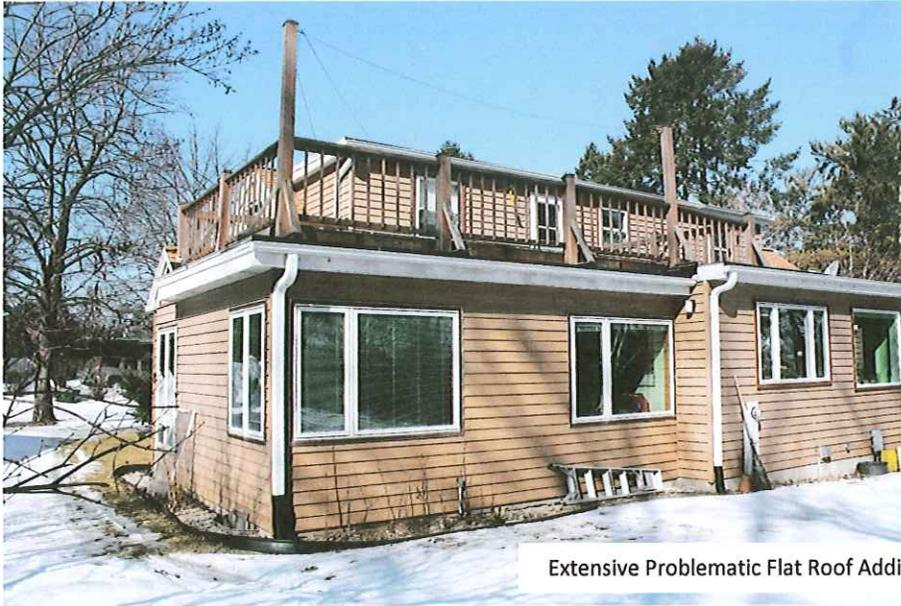
Extensive Problematic Flat Roof Additions over crawl spaces line the entire East face of the original structure
