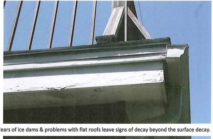
Years of ice dams & problems with flat roofs leave signs of decay beyond the surface decay.
