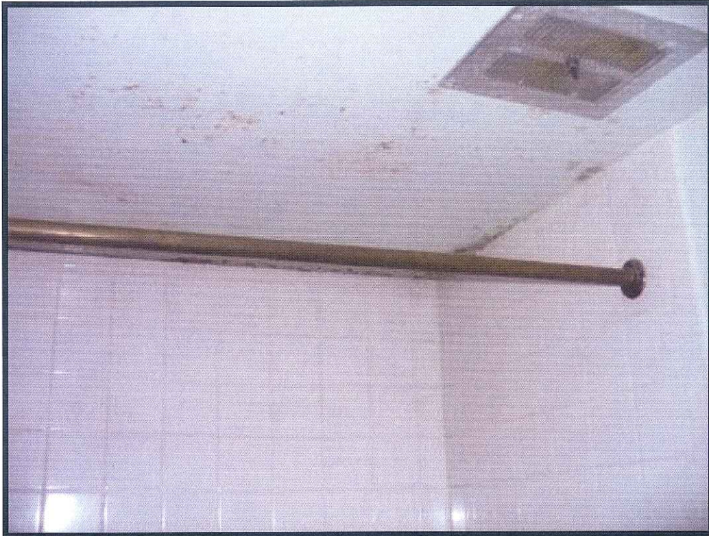
Typical apartment bathroom ceiling
