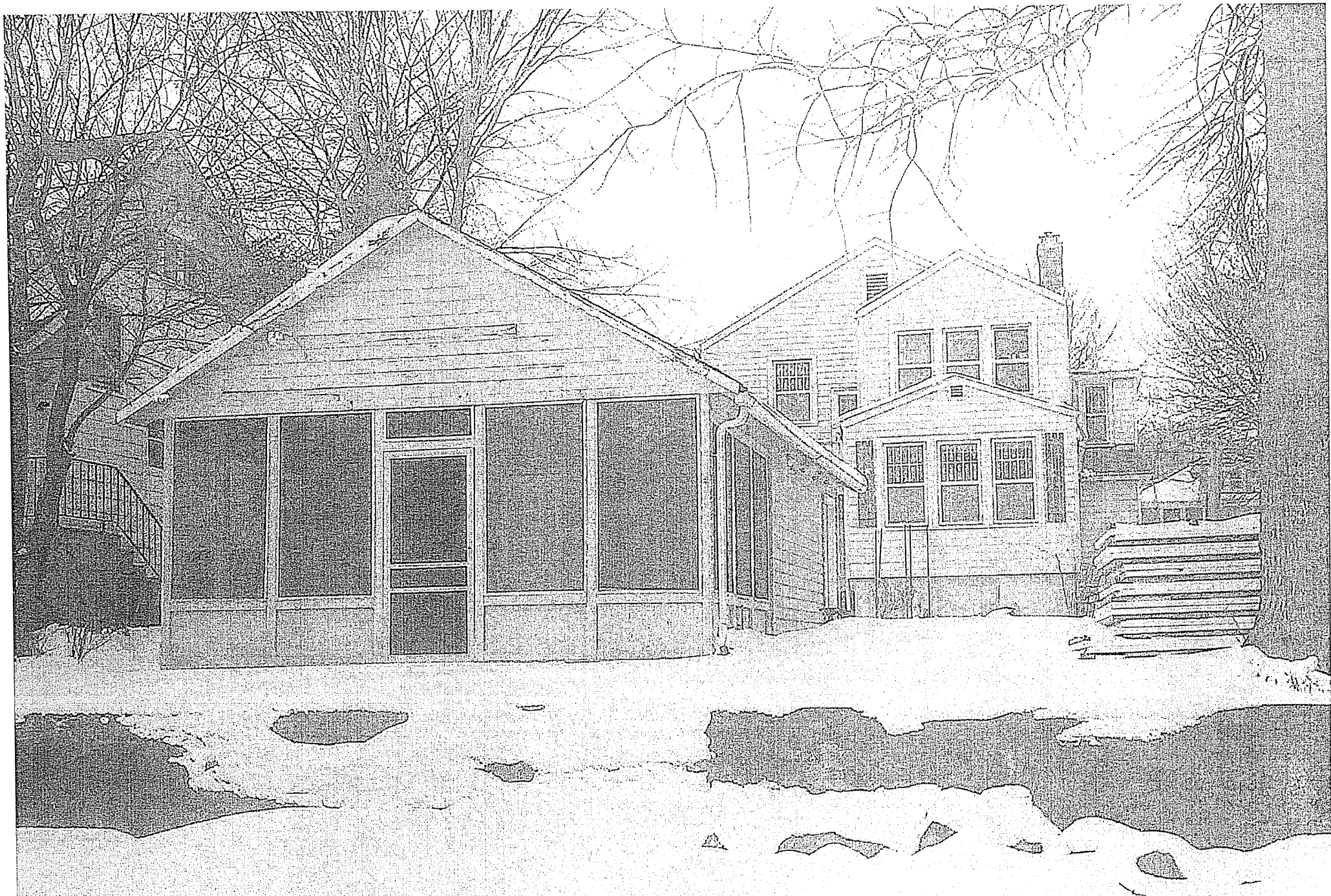
SOUTH (LAKE) ELEVATION. SUBJECT PROPERTY
