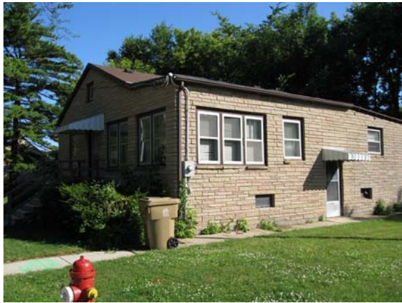
Photo of existing home at 171 Proudfit Street
