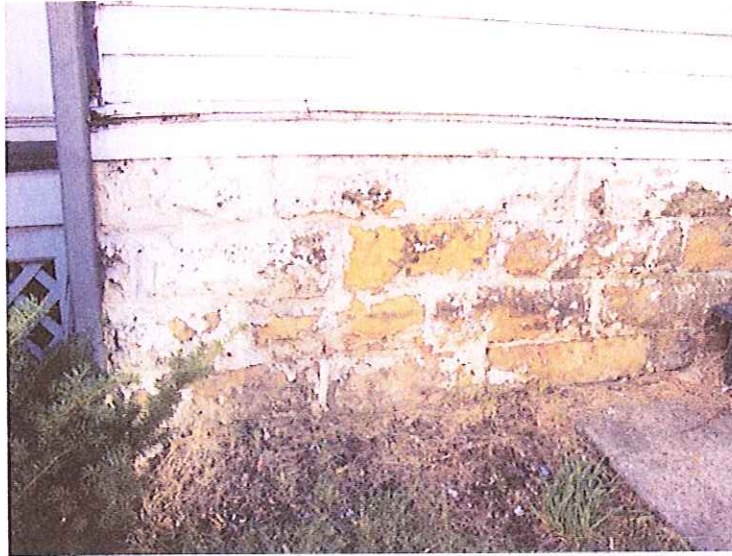
Image of 201 E. Mifflin St. showing the deterioration of the stone masonry foundations walls
