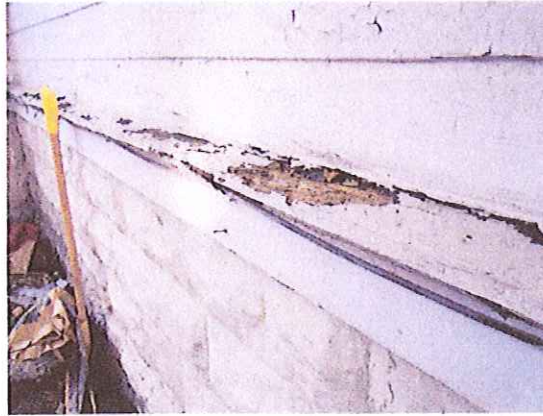
Image showing water infiltration and location of possible damage to framing at the water table trim. East side of 201 E. Mifflin St.
