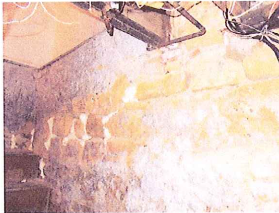
Image showing deteriorated stone foundations and spray insulation filler at 19 N. Webster St.
