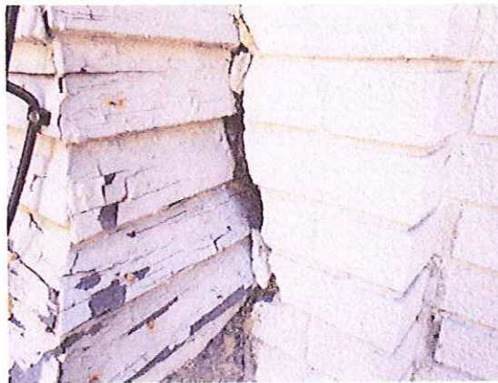
Image showing the path of water infiltration into framing areas at the porch and house intersection. 19 N. Webster St.
