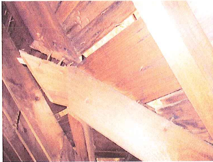
Image showing damaged roof framing at dormer framing. 17 N. Webster St.
