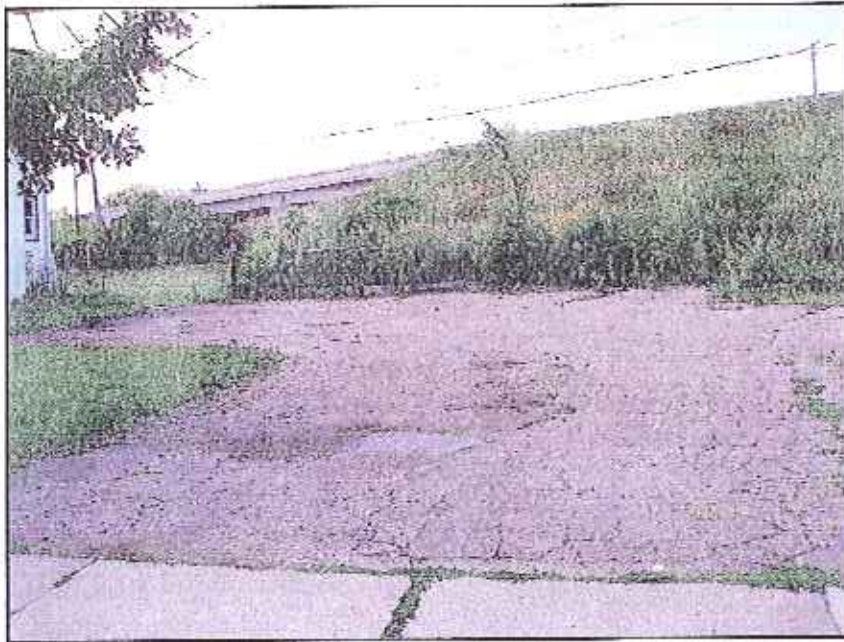
4 Car Parking Lot, facing Southwest
