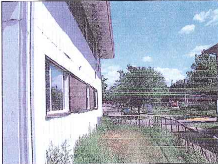
Side Yard, Facing East
