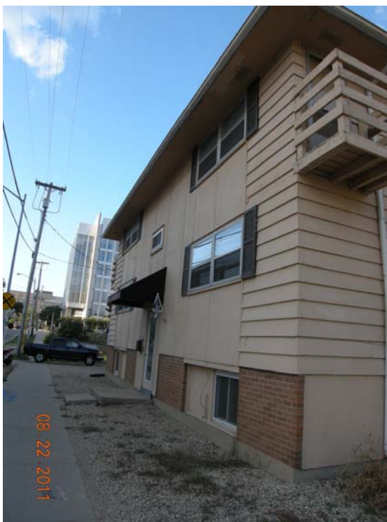
Exterior, west façade
