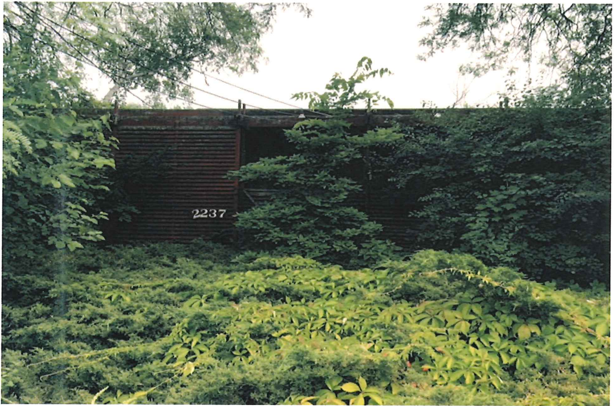
Demolition Permit Photos -2237 Sherman Avenue
