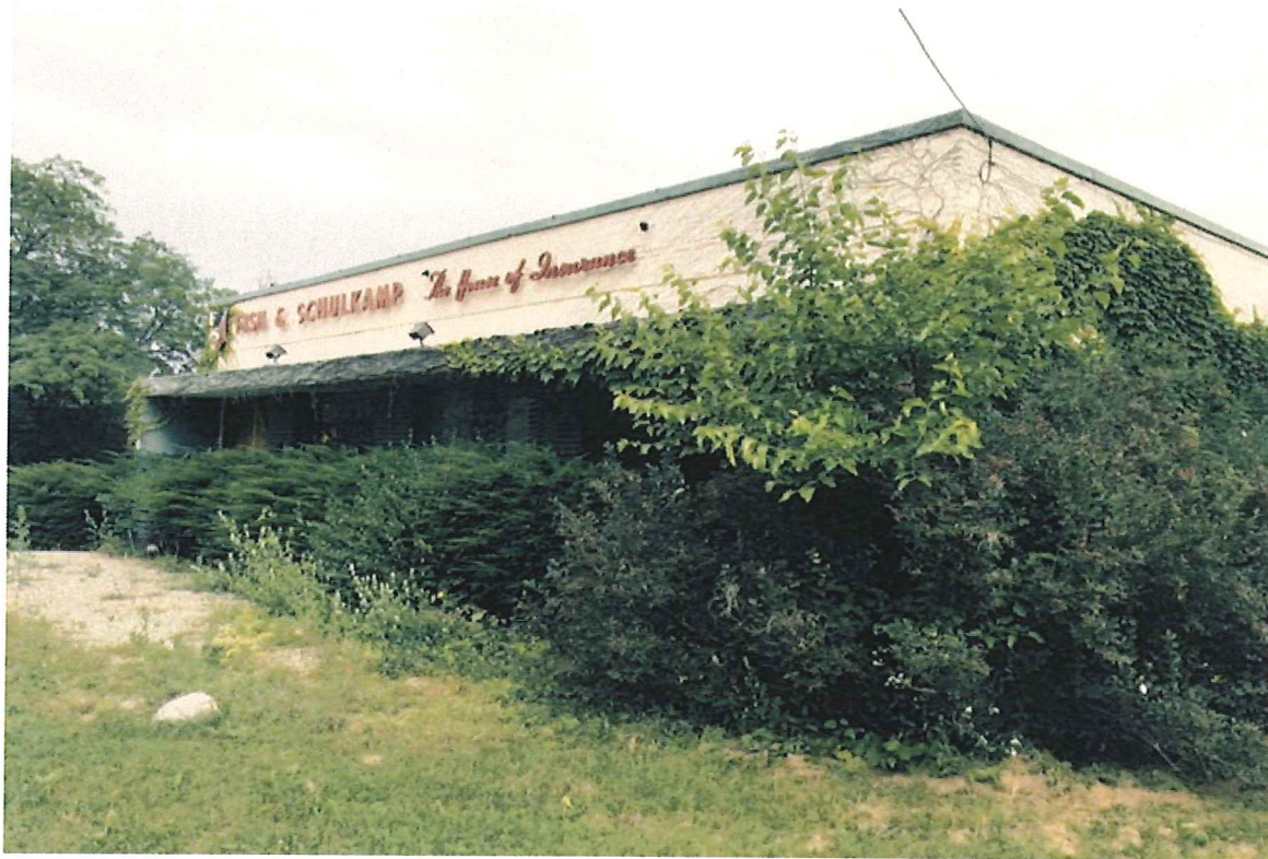
Demolition Permit Photos – 2117 Sherman Avenue
