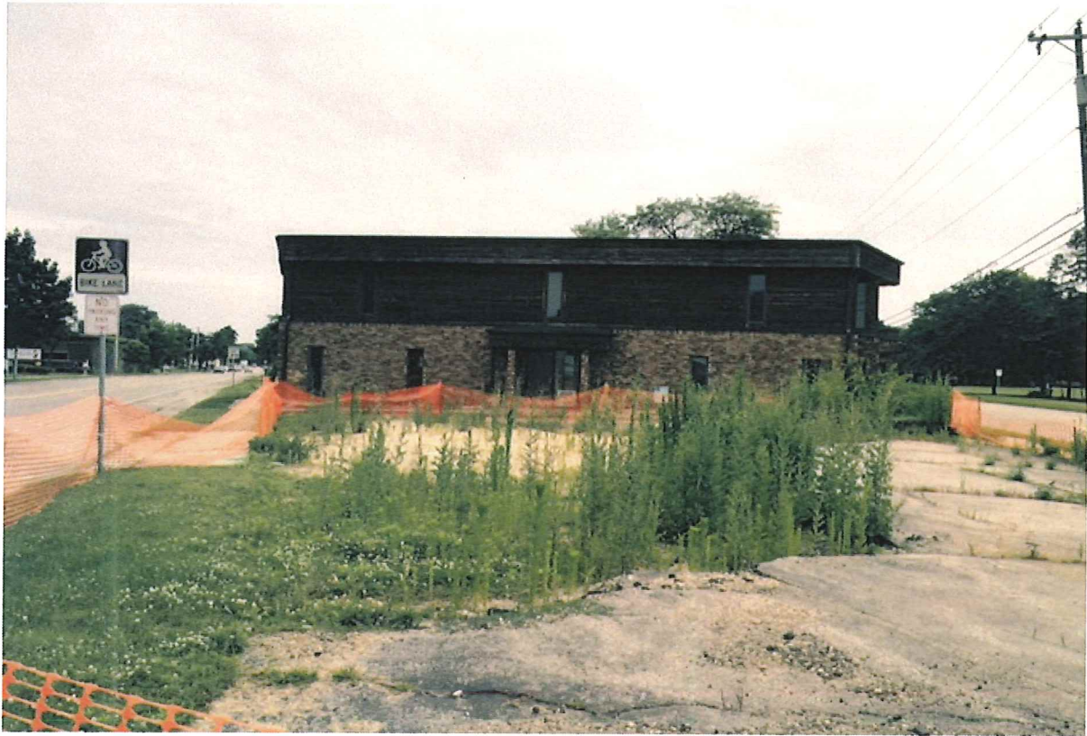
Demolition Permit Photos 2249 Sherman Avenue
