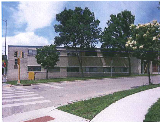
Exterior - East Elevation
