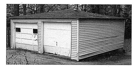
We are proposing to replace this garage at 2830 Waunona Way. These photos are current (11/18/07) and undoctored. We are planning to rebuild the walls to the existing height (8') and to make the roof pitch match the existing house (between a 10/12 and an 11/12). We plan to reuse most of the existing foundation but will need to move the west foundation wall so that it conforms to current setbacks. Probelms with the existing garage:
