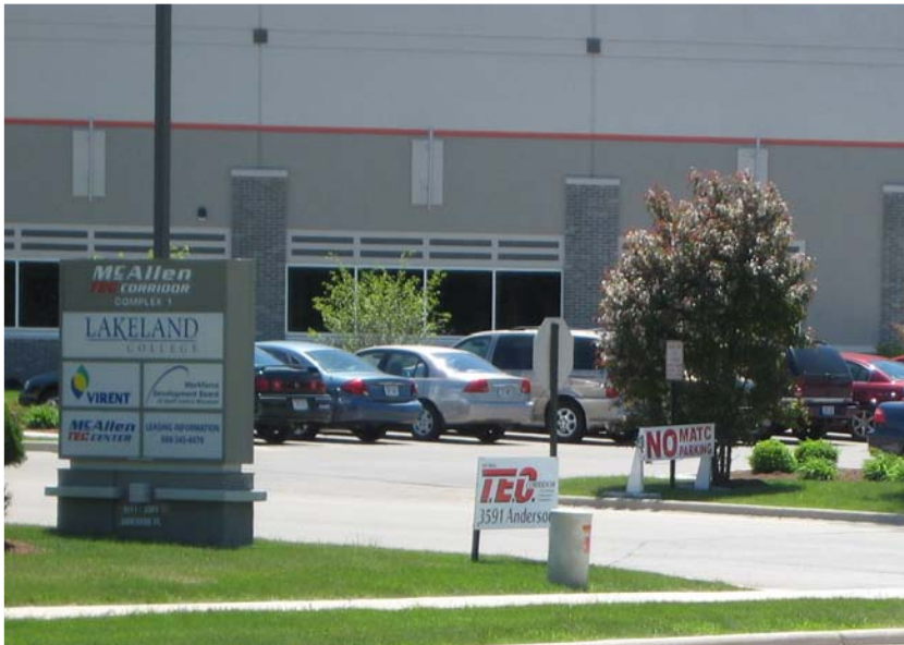
Students often illegally park in adjacent private parking lots.
