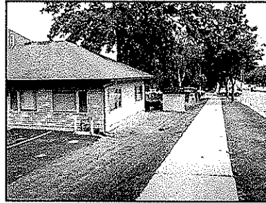
SOUTHWEST CORNER OF EXISTING BUILDING
