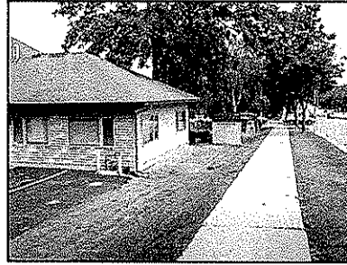
SOUTHWEST CORNER OF EXISTING BUILDING
