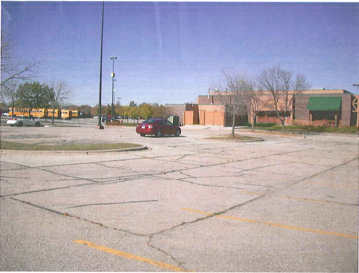
6) View – north, from Mall entrance drive
