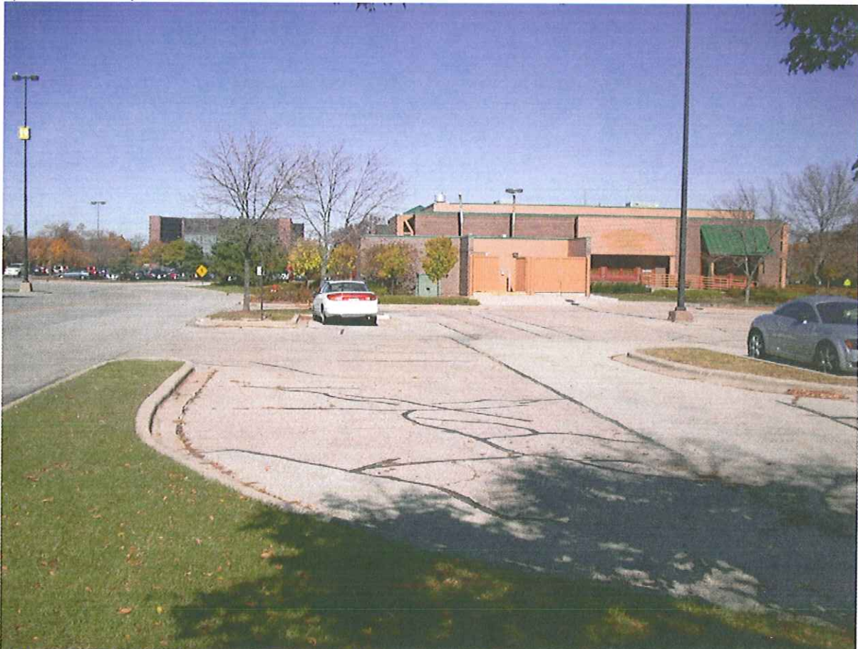
7) View – north, from Mall Ring Road @ Mall Entrance Drive
