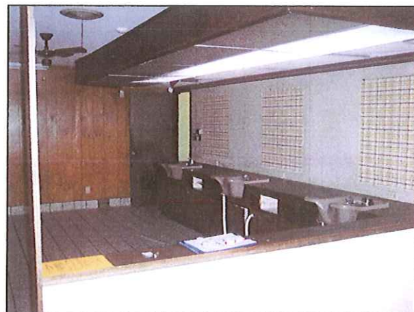
TENANT TO BE DEMOLISHED
