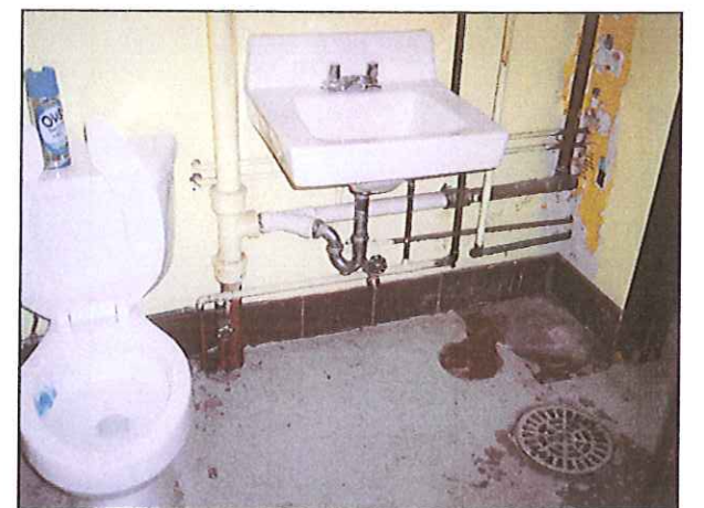
TENANT TO BE DEMOLISHED
