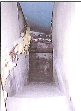
STAIR TO PARTIAL LOWER LEVEL
