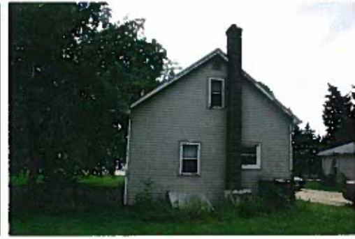
IMG_0967 4706 North Side
