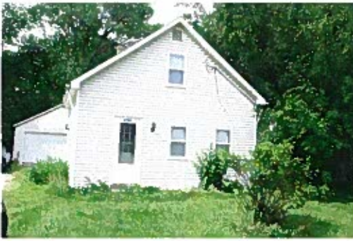
IMG_0965 4706 South Side
