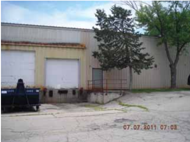
5107 UNIVERSITY AVENUE, FORMER "LOWER WAREHOUSE"
