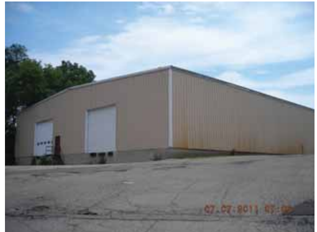
5111 UNIVERSITY AVENUE, FORMER "UPPER WAREHOUSE"
