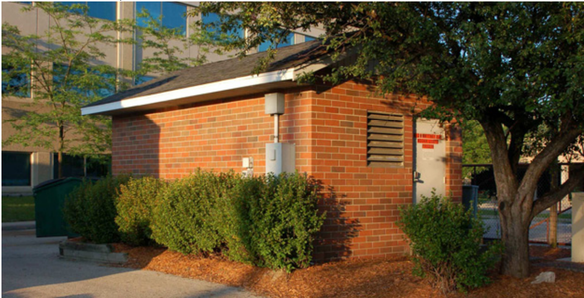
Easement, "AT+T Utility Shed"
