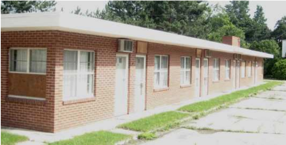
5119 University Avenue, "Quonset Hut"
