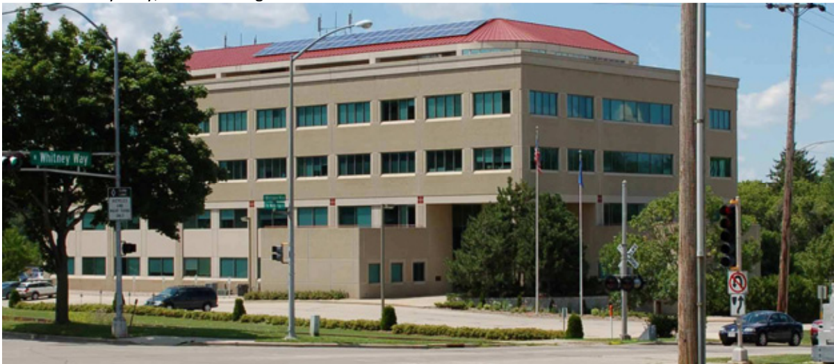
610 N. Whitney Way, "PSC Building"
