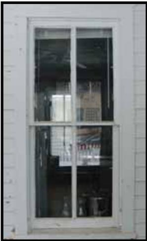
The original window casing and crown molding will be reproduced on the new exterior. The new high-efficiency double-hung fiberglass windows will maintain the 2-over-2 muntin layout found on many of the existing windows in the house.
