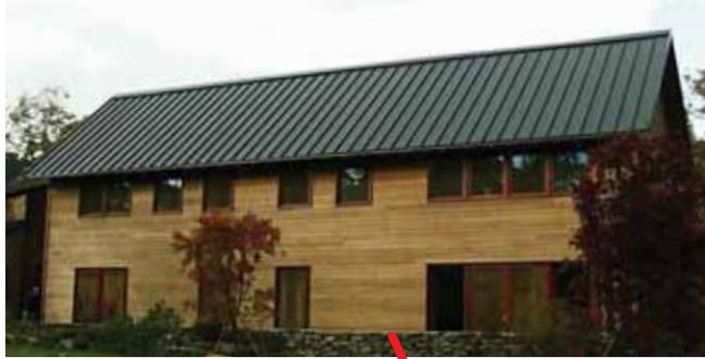
The existing roof and walls of the structure will be wrapped in rigid insulation
