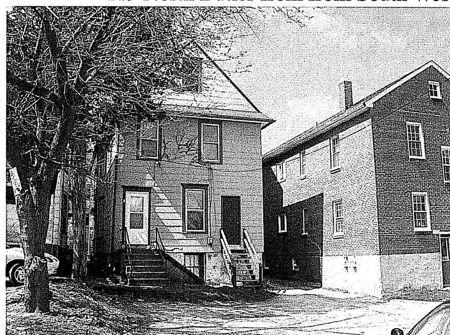
119 North Butler from from South East
