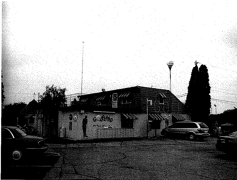
Existing Vitense Building to be Demolished
