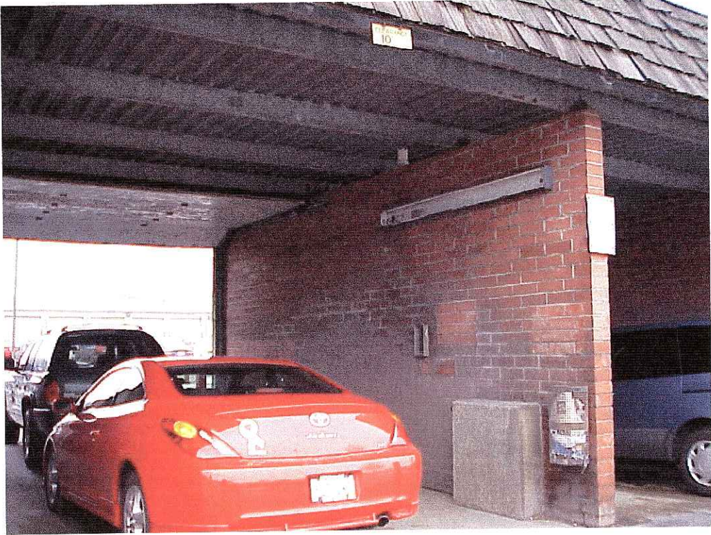
Existing Building – Physical Condition
