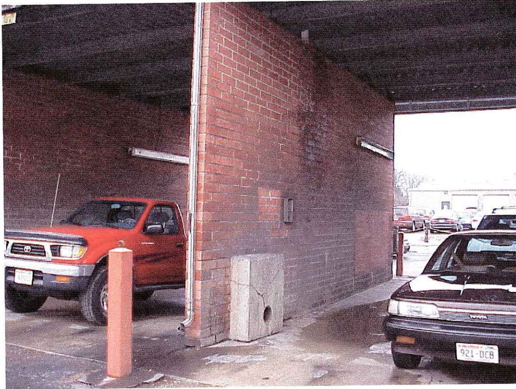
Existing Building – Physical Condition
