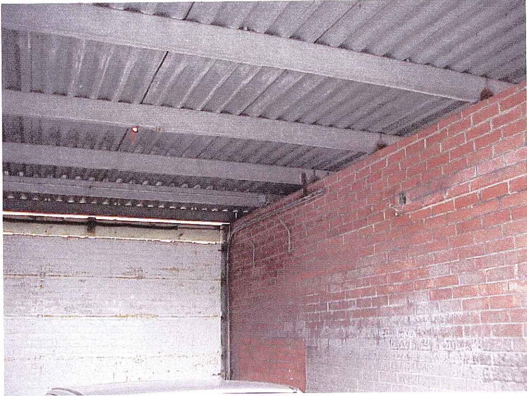
Existing Building - Physical Condition
