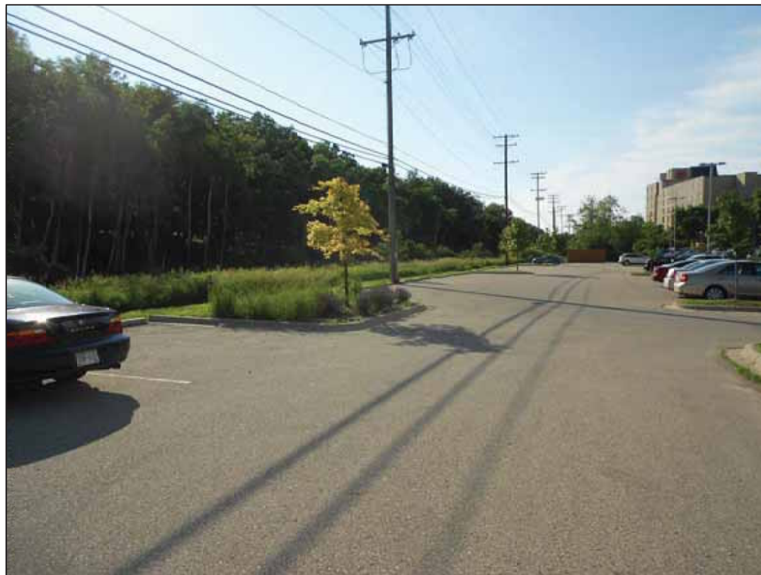
SITE LOOKING NORTH AT EXISTING PUMP HOUSE
