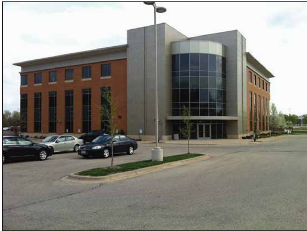
EXISTING 660 JOHN NOLEN DRIVE OFFICE BUILDING
