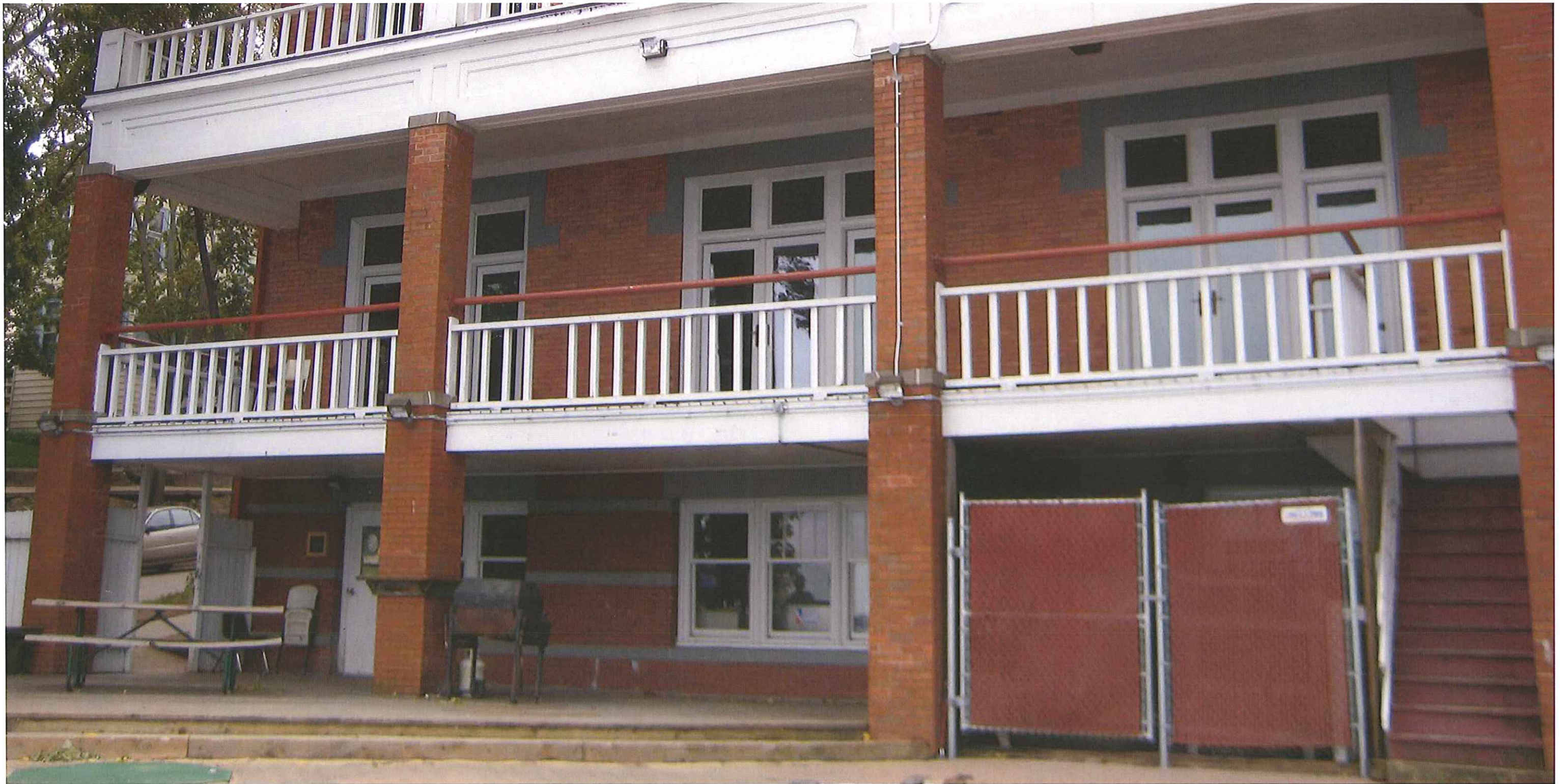
Current Conditions - Exterior - Lakefront Facade
