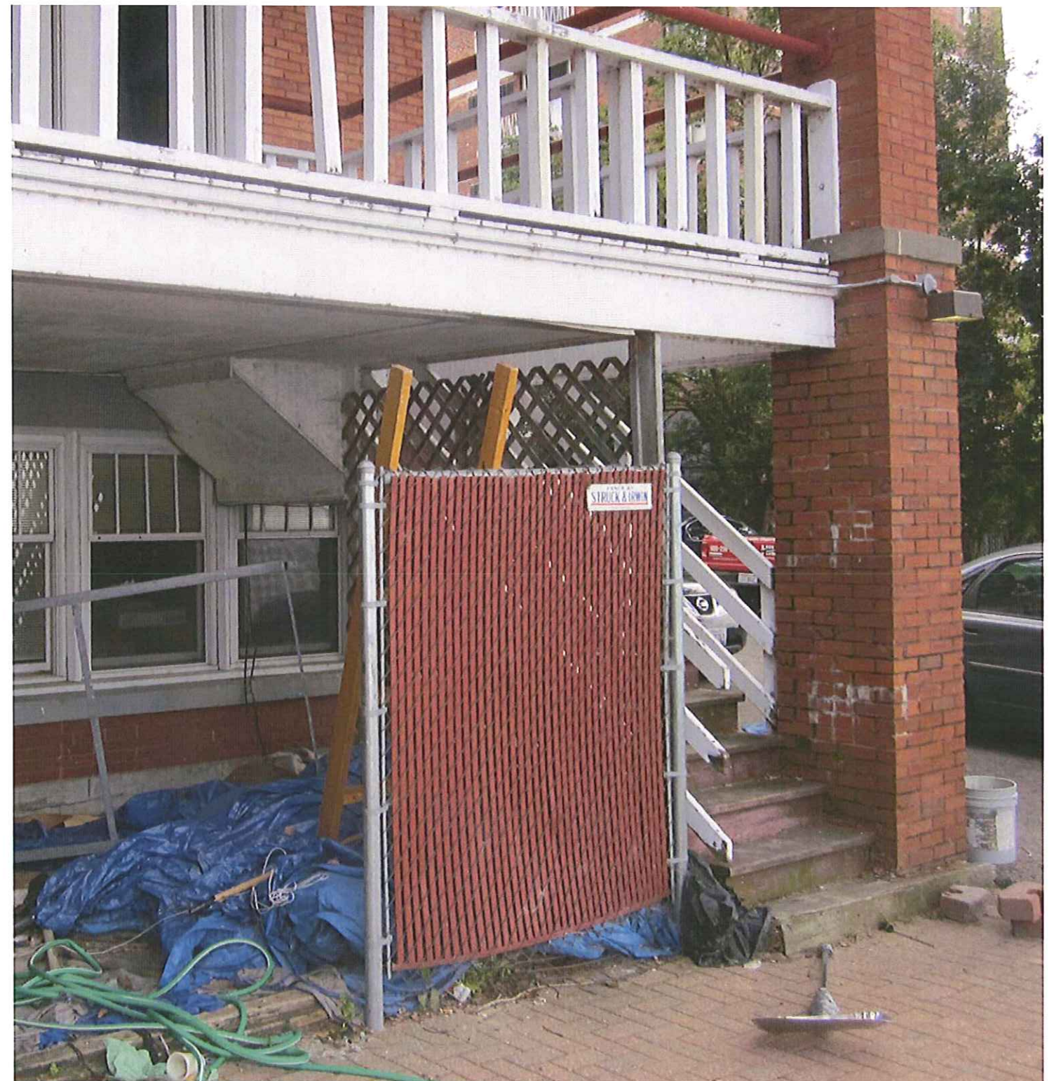
Current Conditions - Exterior - Lakefront Facade
