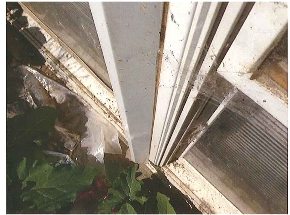
Current Conditions - Windows
