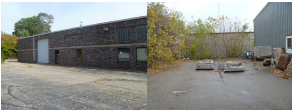
Exterior photographs of existing loading zone and rear lot
