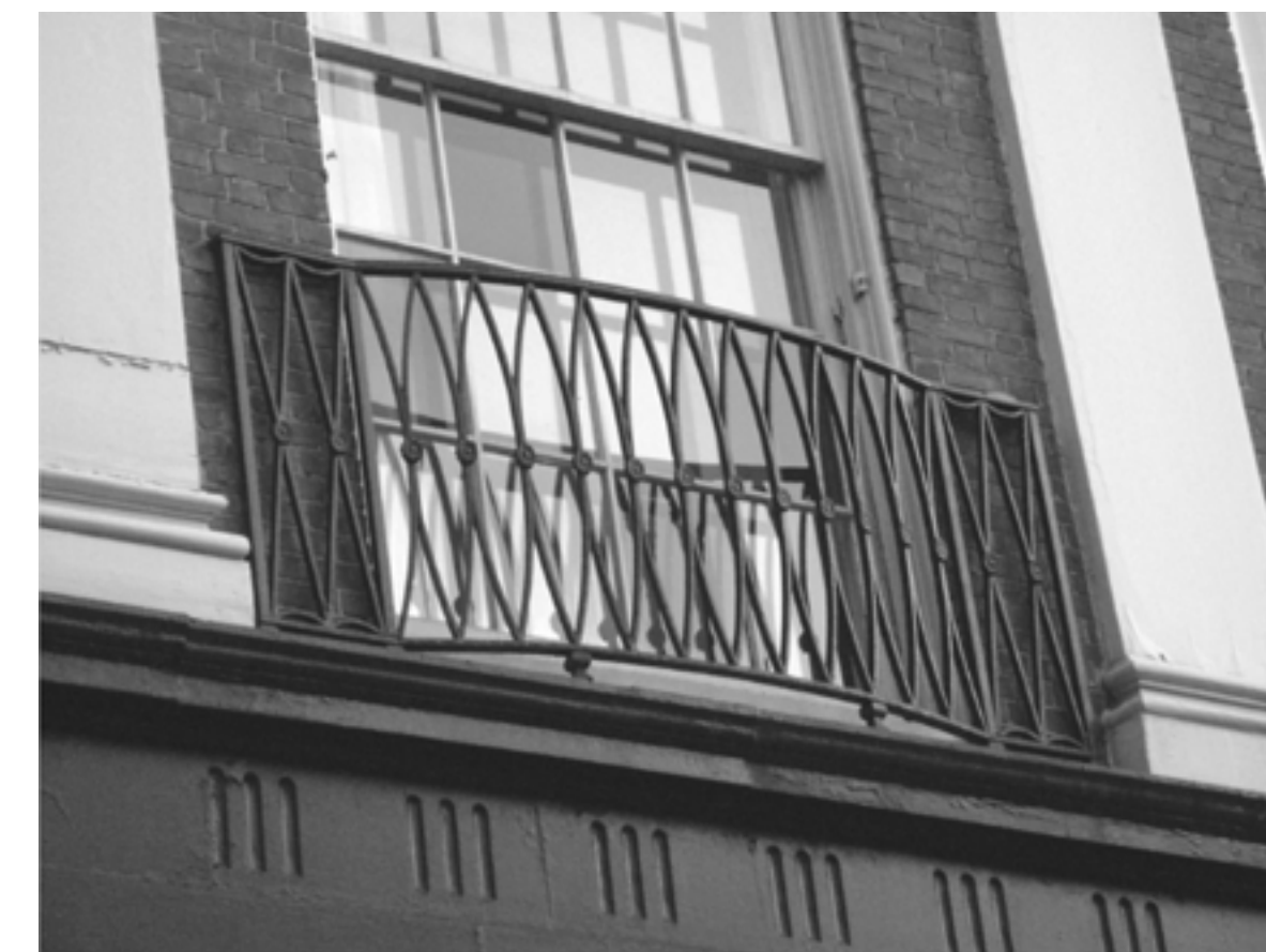
2 Painted Metal Railing Reference Image SCALE: N.T.S.
