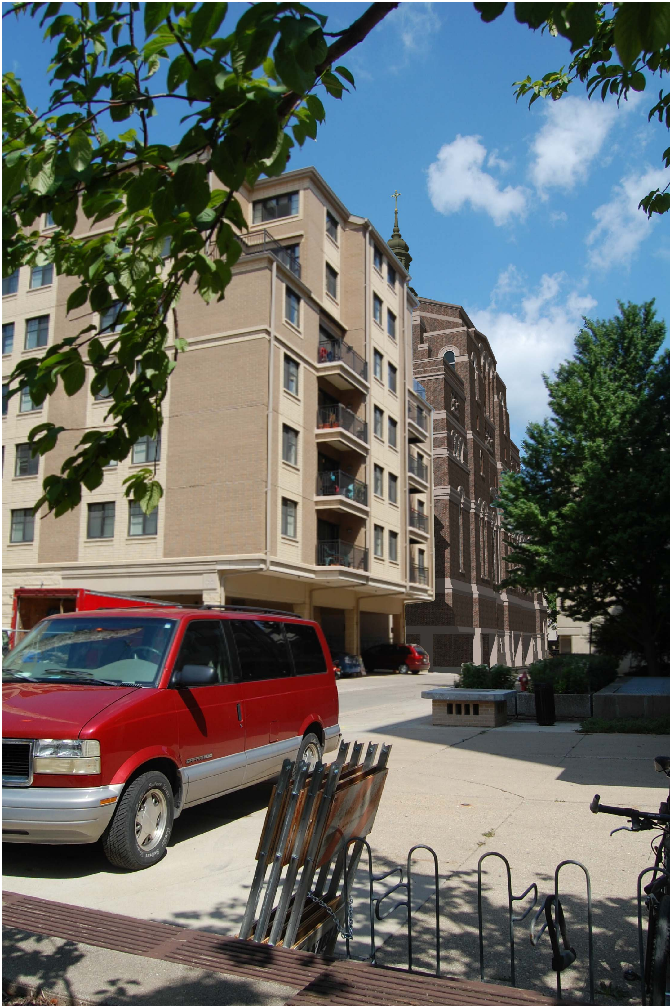
VIEW FROM SOUTH FITCH COURT
