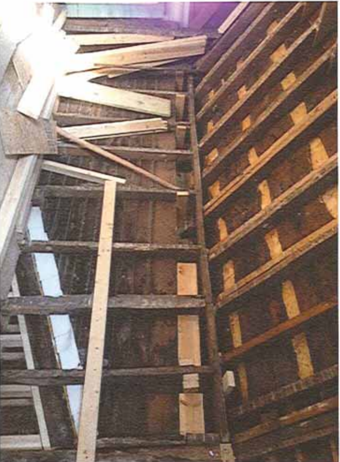
Image 36: Single sill plate supporting roof joists.
