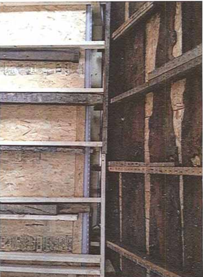
Image 35: Single sill plate supporting roof joists.
