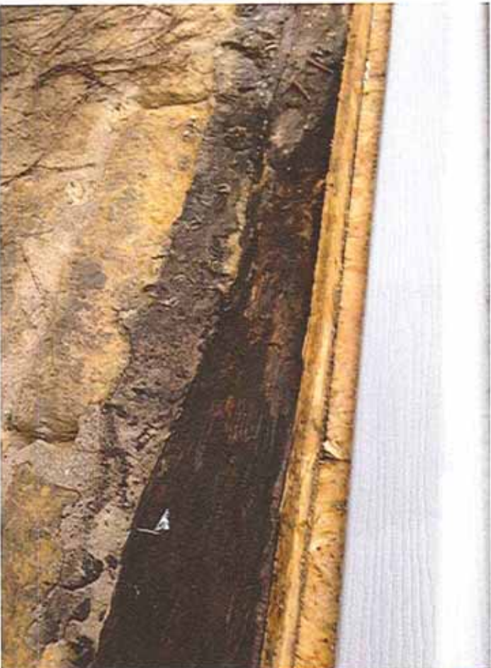
Image 9: Rolling wood bearing on the foundation wall.
