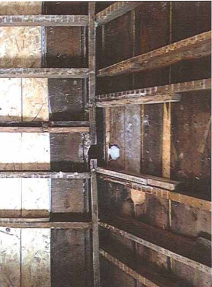
Image 34: Single sill plate supporting roof joists.
