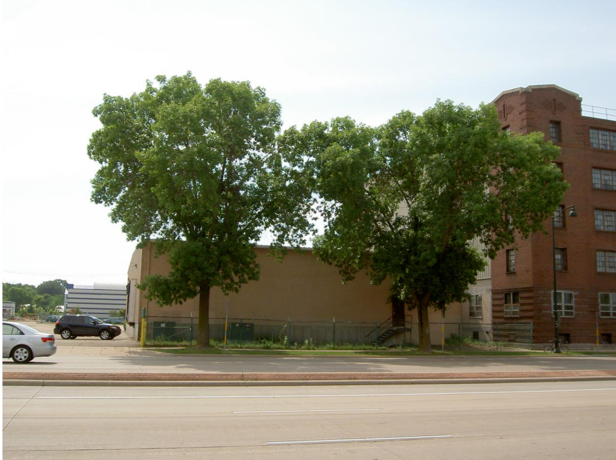
905 East Washington Avenue – Metal Building
