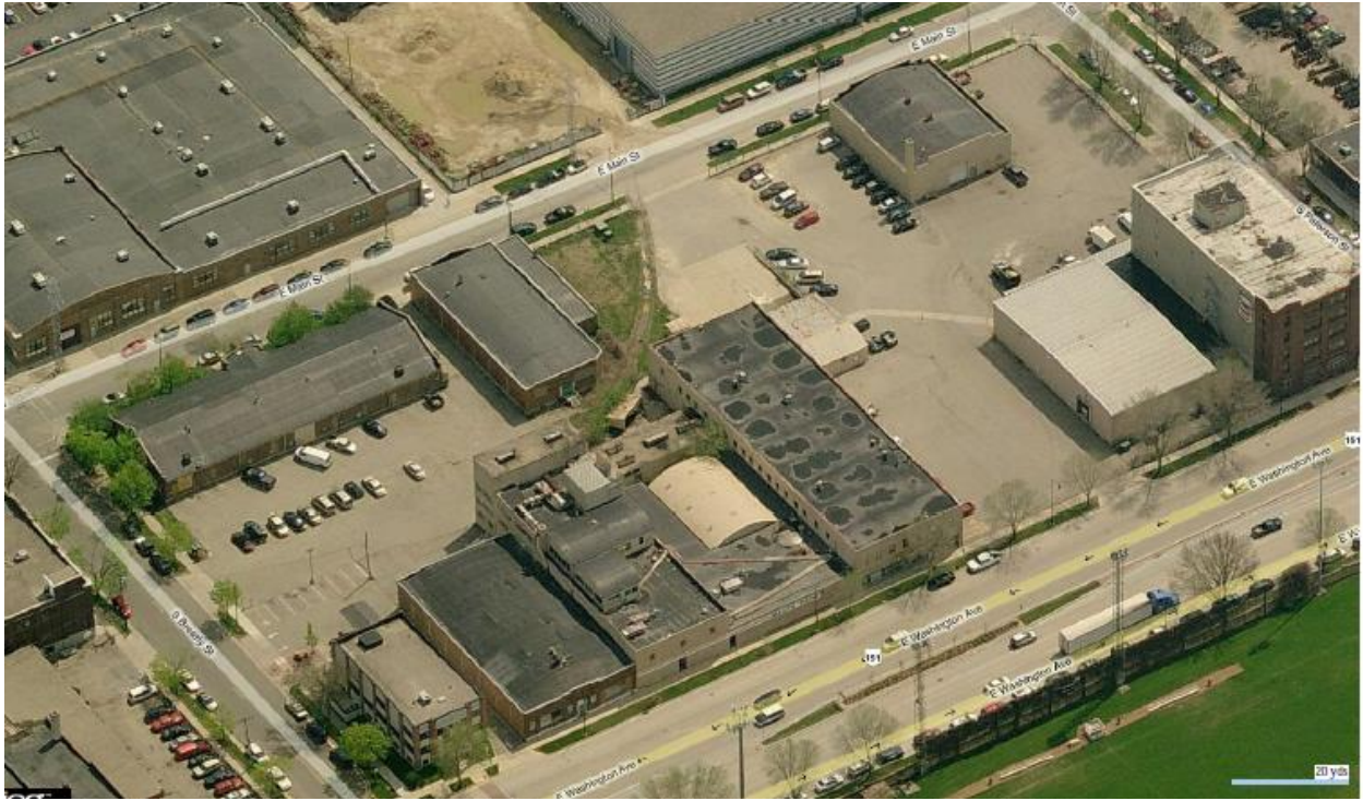
Aerial View from North East
