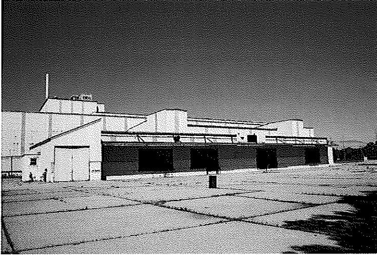
Storage Building with Granulation Building in background
