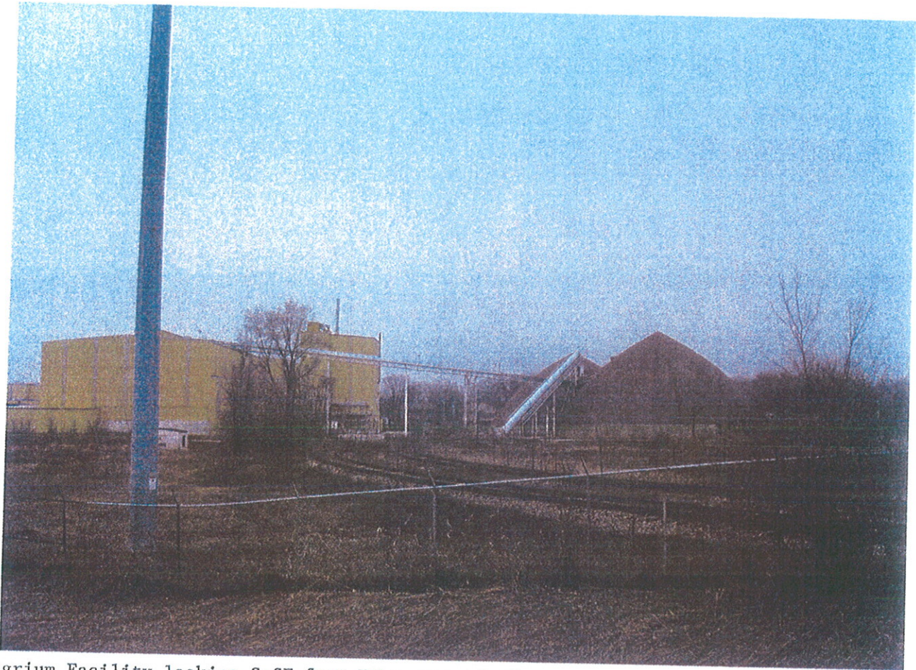
Agrium Facility looking S-SE from NW corner of site
