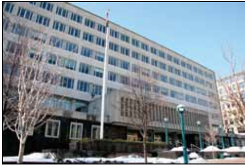
Central District Station/Administrative Offices
