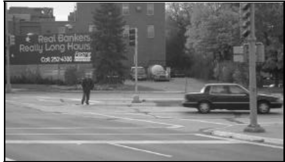
Refuge islands allow pedestrians to cross traffic in each direction of travel separately.
