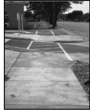
The curb ramps across the main entrance into Westgate on Whitney Way could be improved to provide a straighter line of travel for pedestrians.
