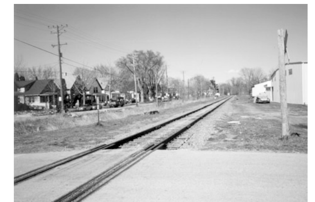
Rail corridor at Second Street and East Main Street
